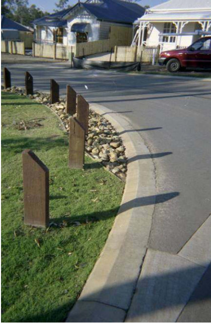
Figure 6: Example of a swale protected by bollards
