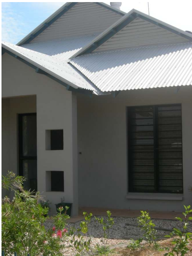
Figure 31: Darwin house with a gravel infiltration area
