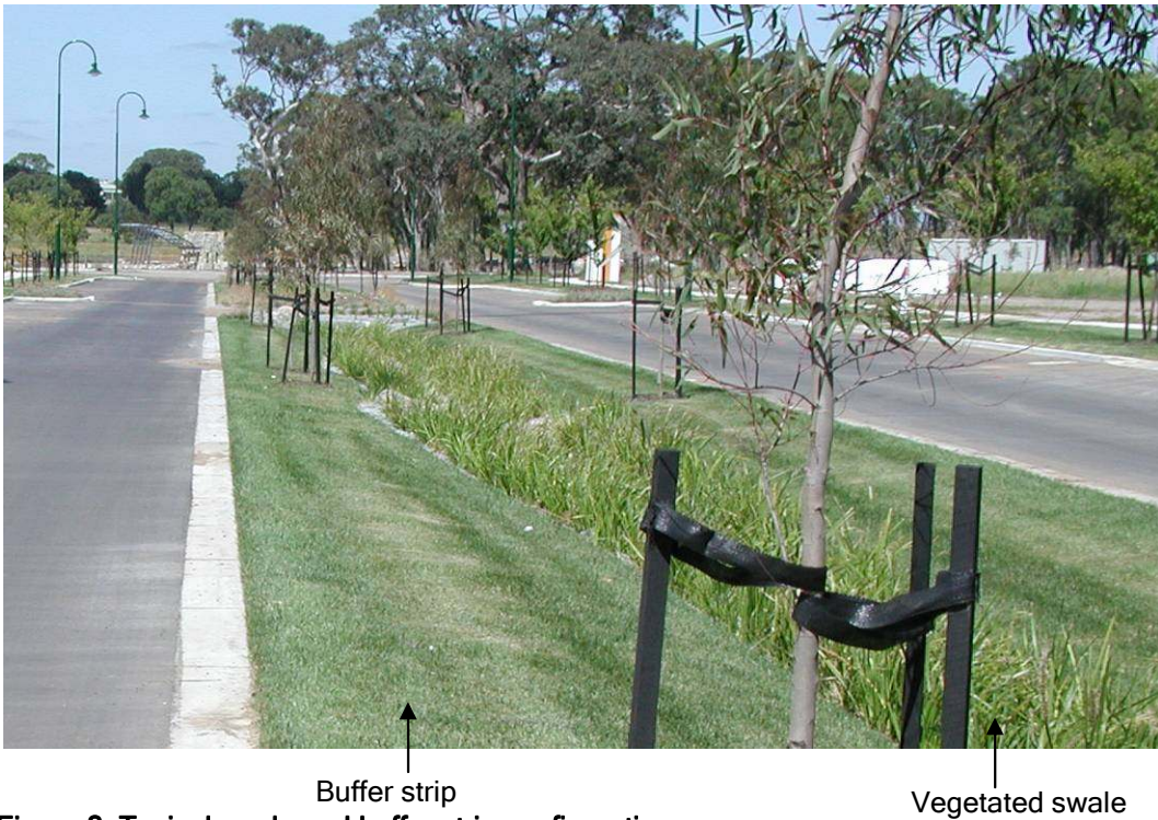
Figure 8: Typical swale and buffer strip configuration
