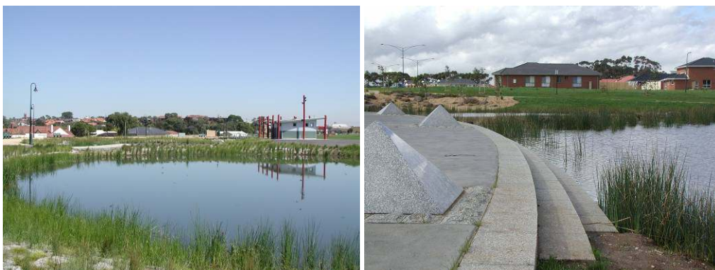
Figure 5: Ponds at All Nations Park, Northcote Victoria (left) and Cairnlea Estate, Victoria (right)
