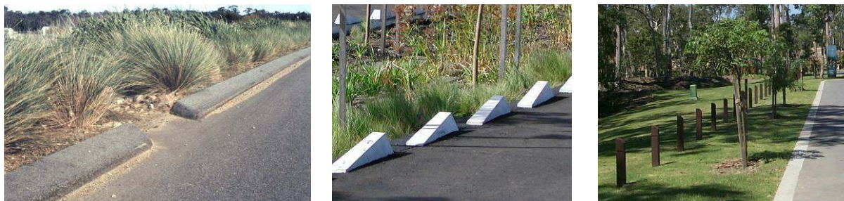
Figure 12: Different arrangements for delivering water to a swale and preventing vehicular access
