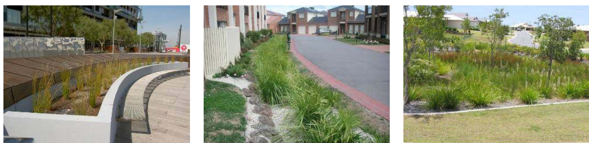
Figure 14: Examples of bioretention systems in planter boxes, in the streetscape, and in parks
