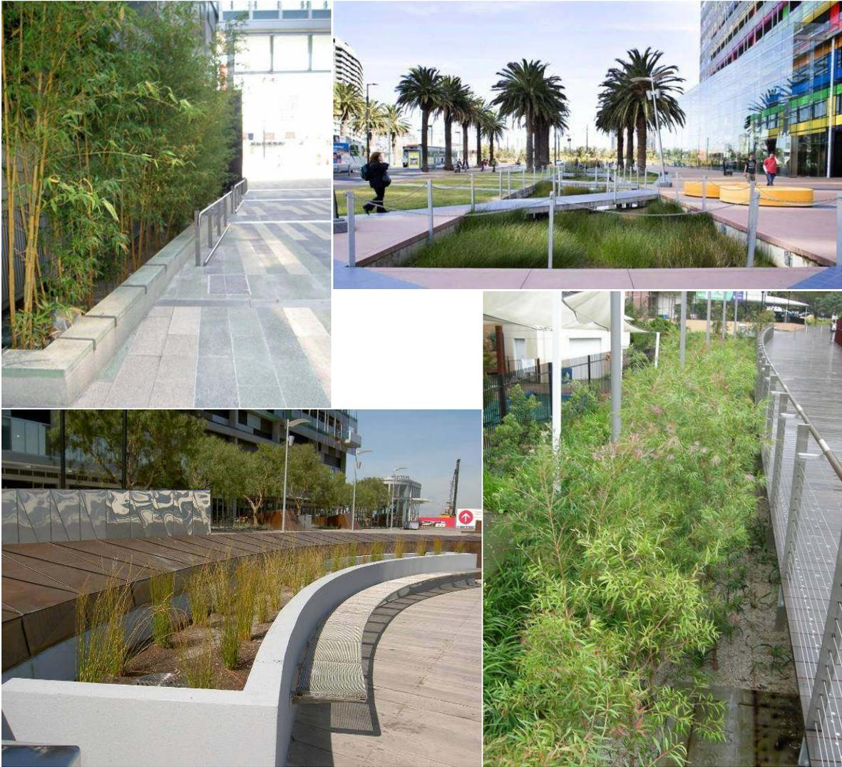
**Figure 4: Stormwater treatment systems in plazas, walkways and building forecourts**
